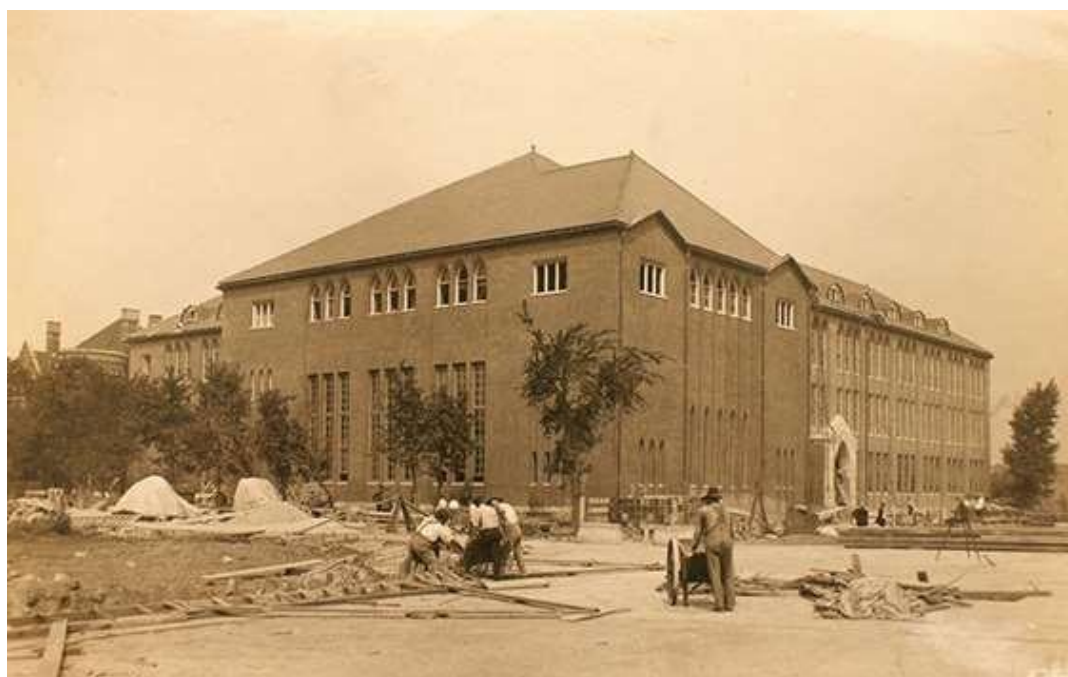
The monumental main building (1922) and the subsequent additions (1955) were both designed by Barry Byrne (1883-1967), a Chicago native and one of Franklin Lloyd Wright's four best known students (sumber: http://www.aicusa.edu )
